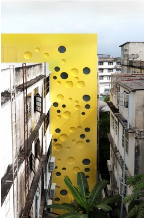
The Utility Stick. Courtesy: Lin Ho/Spark Architects/TMB Bank
